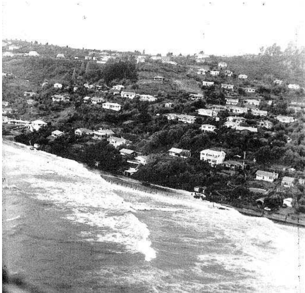
Figure 4-4: Aerial photograph of wave set-up and run-up at Rocks Road taken at ~13:00 during the 19 March 1957 storm. [Supplied by M. McGuire, Port Nelson].
