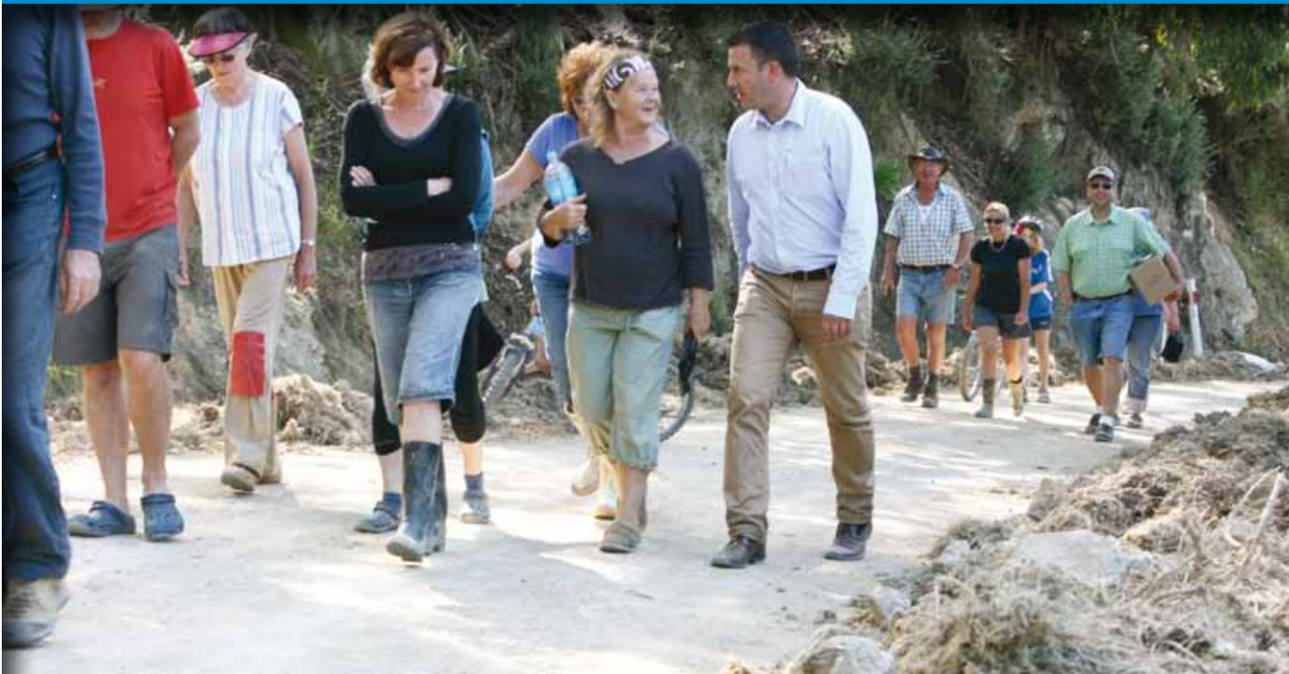
Nelson Mayor Aldo Miccio meets with Cable Bay residents to view the damage.
