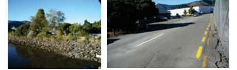
② River edge dominated by carparking, vehicle movement. River obscured by dense edge planting.
