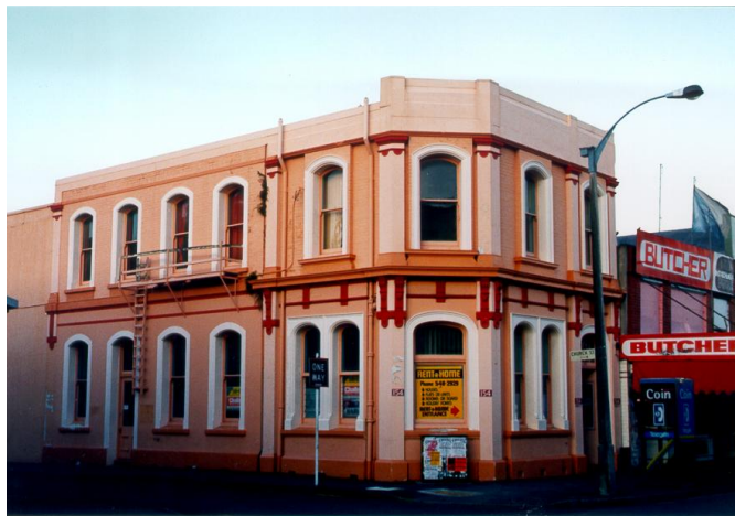
Expression of floors and columns scales a two-storey building to the street and neighbours...
